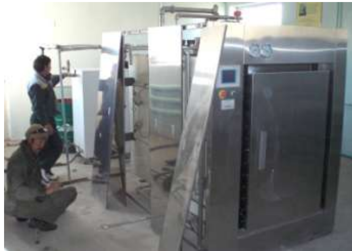
Pic: Installation of autoclaves (Ulaanbaatar, Mongolia) © ETLog Health, 2010
