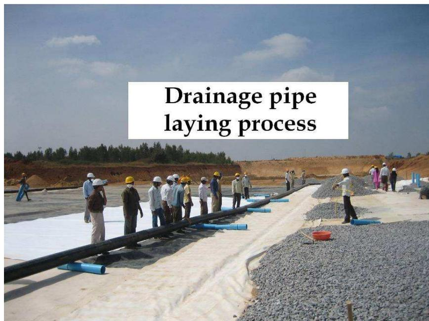
A surface sealing system is provided on the top of the waste fill at the end of each construction phase, to control the leachate production by reducing the ingress of rain into the fill. The surface sealing system comprises a compensation layer, mineral sealing layer, geomembrane, geotextile, drainage and recultivation layer.
