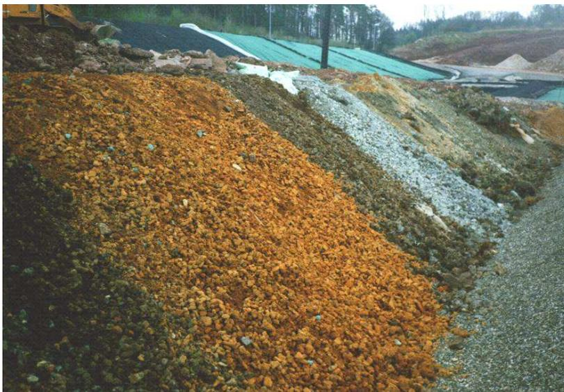
Fig. 51: Different types of residues from physico-chemical treatment containing dangerous substances, disposed on an above-ground hazardous waste landfill
