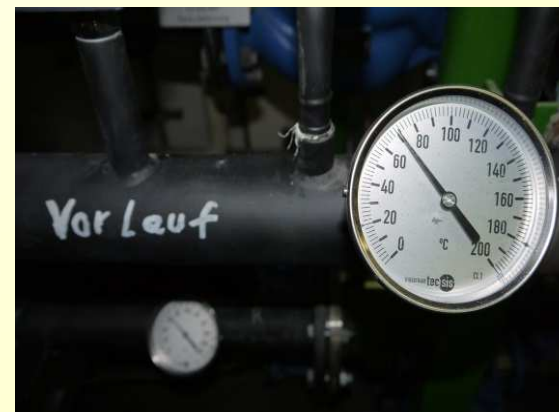
Internal heat consumption of the plant approx. 80.000 MWh
