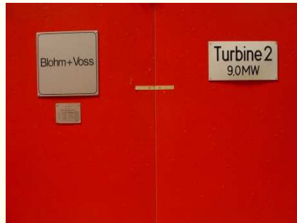
Power generation 120.000 MWh total output 95.000 MWh export to the national grid
